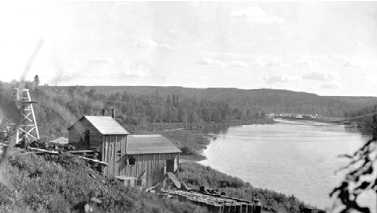
Fig. 20 D. S. Pasternack, Oil Extraction Plant - Clearwater River Plant . The plant processed 800 tons of oil sands in the summer of 1930, and yielded over 75 tons of bitumen (Ferguson 54).
