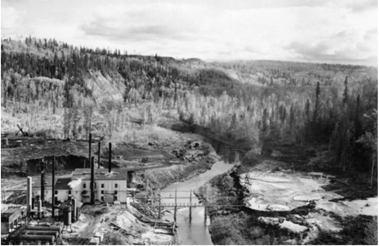
Fig. 31. George Sherwood Hume, Abasand Plant alongside Horse River . Note cribs for waste sands.
