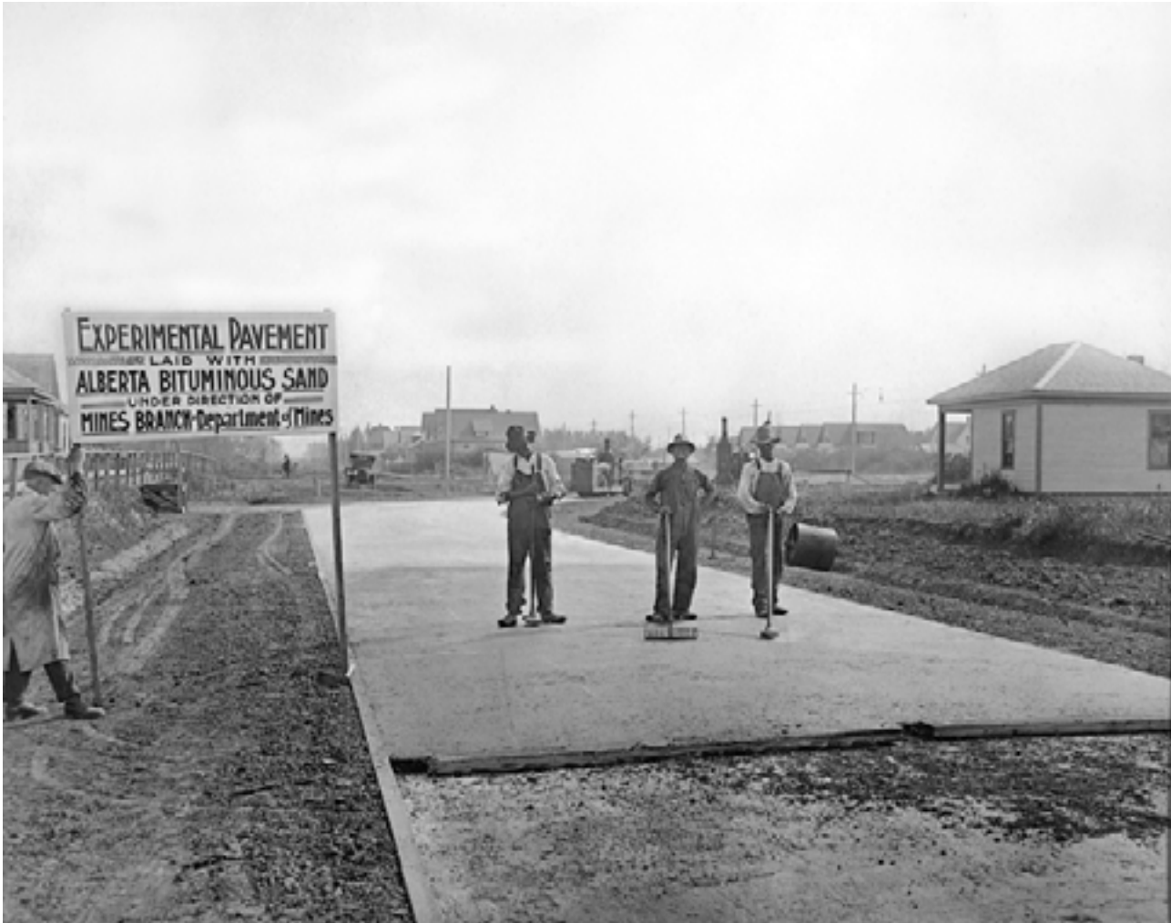
Fig. 23 Robert Fitzsimmons, Experimental Pavement Laid with Alberta Bituminous Sand under Direction of Mines Branch, Department of Mines.
