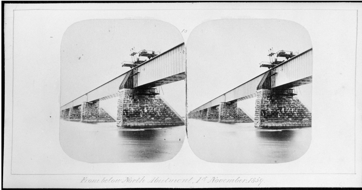
Fig. 2. Victoria Bridge under construction, from below North Abutment, 1859.
