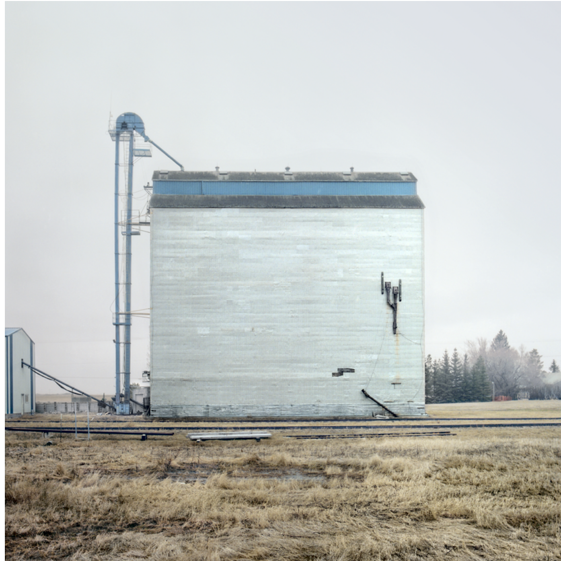
Fig. 7. Saltzman, "Photo 9", trans.plant
