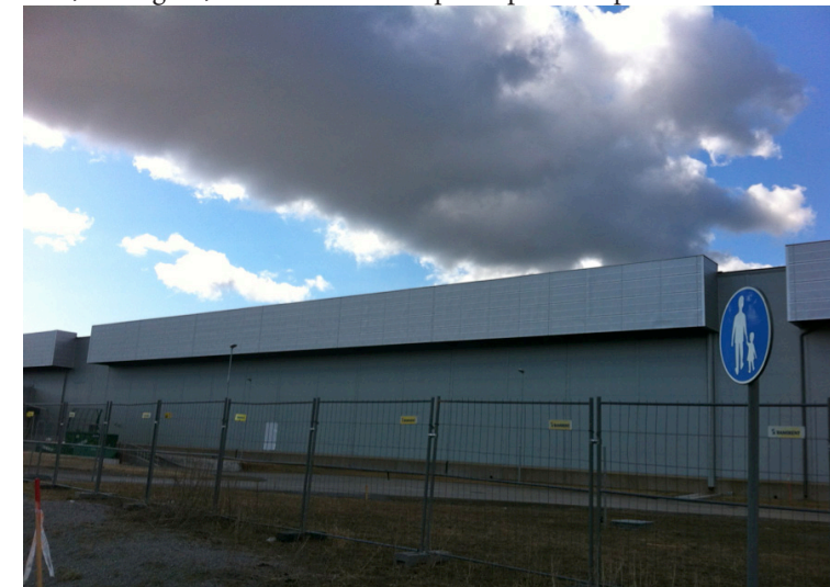
Figure 3. Facebook's first data centre building in Luleå, photographed by author, April 2014.
