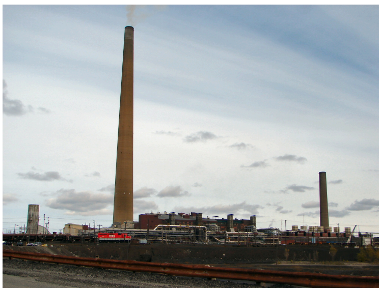
Figure 10: Inco Nickel Smelter Superstack, October 2006
