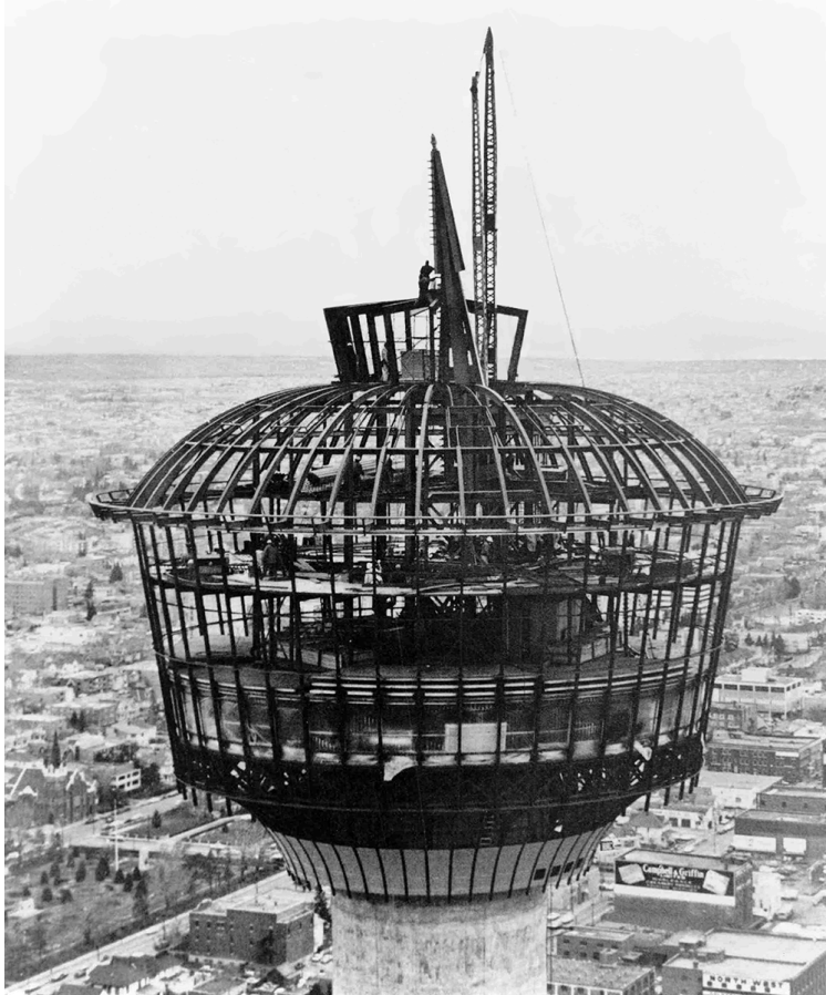
Figure 4: Calgary Tower under construction, 1968
