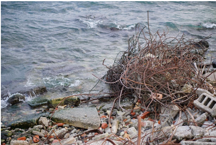
Figure 7: Rebar at Tommy Thompson Park
