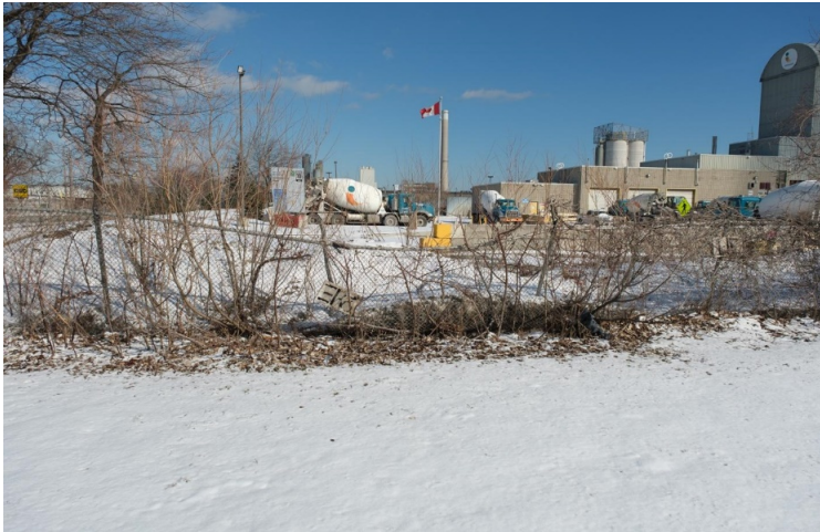
Figure 1: Dilapidated gate and factory next to Tommy Thompson Park
