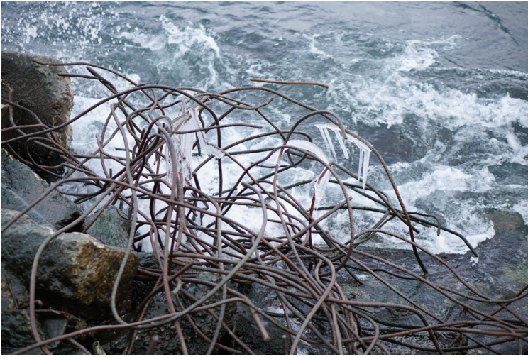
Figure 8: Rebar at Tommy Thompson Park
