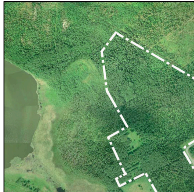
Figure 5. Facebook’s Swedish cloud, seen from above. Buildings to the right include student dormitories and Luleå’s Science Park. (Source: Genomförandebeskrivning/The Description of Implementation, Luleå Municipality 2011 ).
