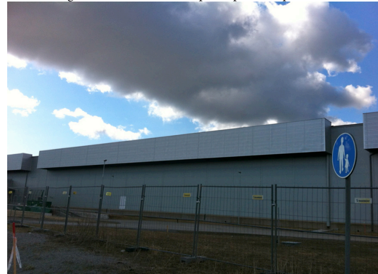
Figure 3. Facebook's first data centre building in Luleå, photographed by author, April 2014.
