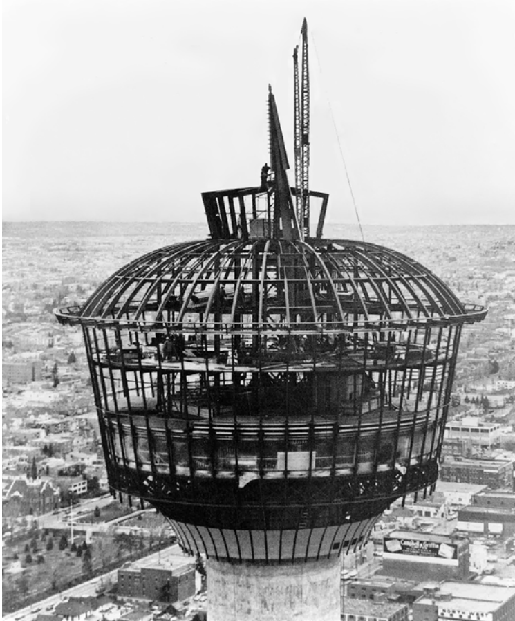
Figure 4: Calgary Tower under construction, 1968
