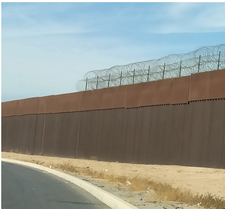
Figure 1: First view of the wall in Mexicali
