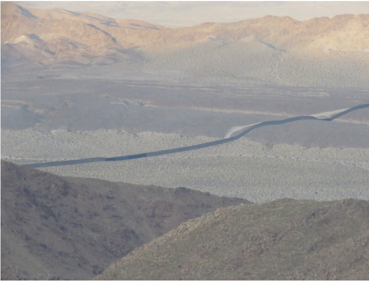
Figure 14: View of the wall from la Rumorosa mountain pass
