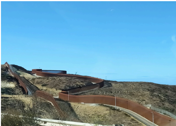
Figure 17: View of the double wall, Tijuana
