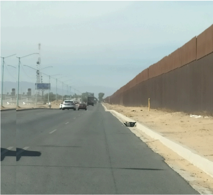
Figure 2: First view of the wall in Mexicali
